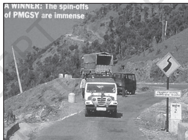
Fig. 7.2 : Road constructed under the Pradhan Mantri Gram Sadak Yojna
