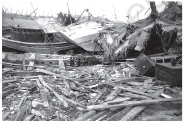
Figure 6.3 : Tsunami Affected Area
