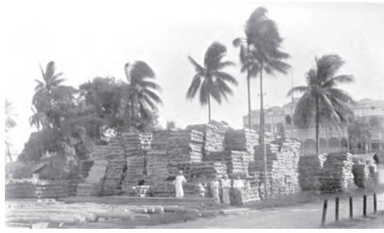
Fig.23 – Indian Munitions Board, War Timber Sleepers piled at Soolay pagoda ready for shipment, 1917.
