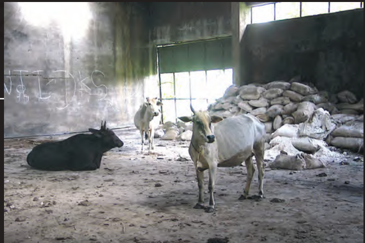
Bags of chemicals lie strewn around the UC plant
