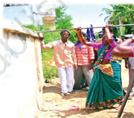
Members of the Safai Karamchhari Andolan demolishing a dry latrine.
