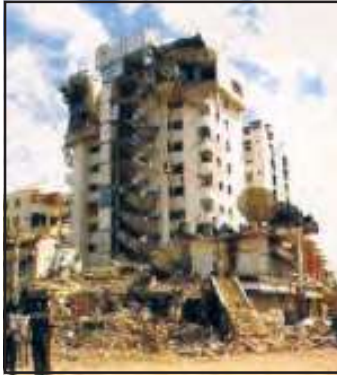
Fig. 3.3a: Destruction caused by an Earthquake in Gujarat
